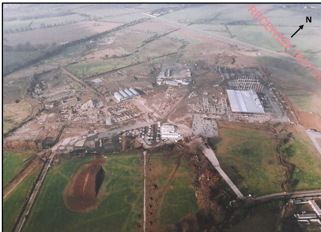
Figure 15.9: Aerial photograph dated February 1996 showing extent of groundworks undertaken as part of the Hewlett Packard Campus development (Source: Tom Kavanagh, Estate Manager, Liffey Business Park).
