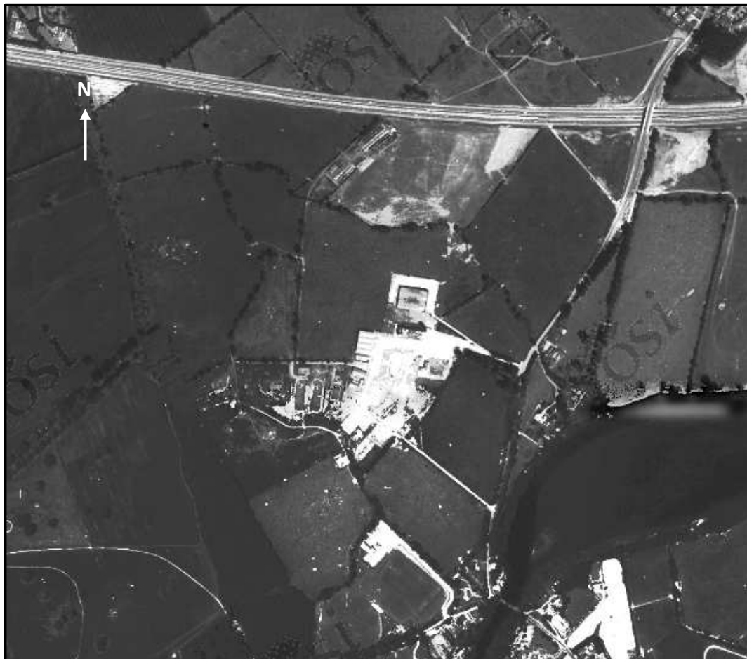
Figure 15.8: Extract from aerial image dated 1995 showing commencement of demolition works at the Irish Meat Packers as part of the Hewlett Packard Campus construction (Source: webapps.geohive.ie/mapviewer ).
